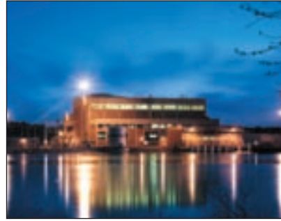
Fort Calhoun Station
