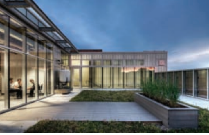
The North High School addition features a green roof.
