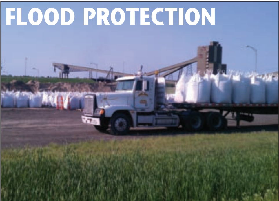
Sandbags weighing 3,000 pounds are being used to create a barrier near Nebraska City Station.
